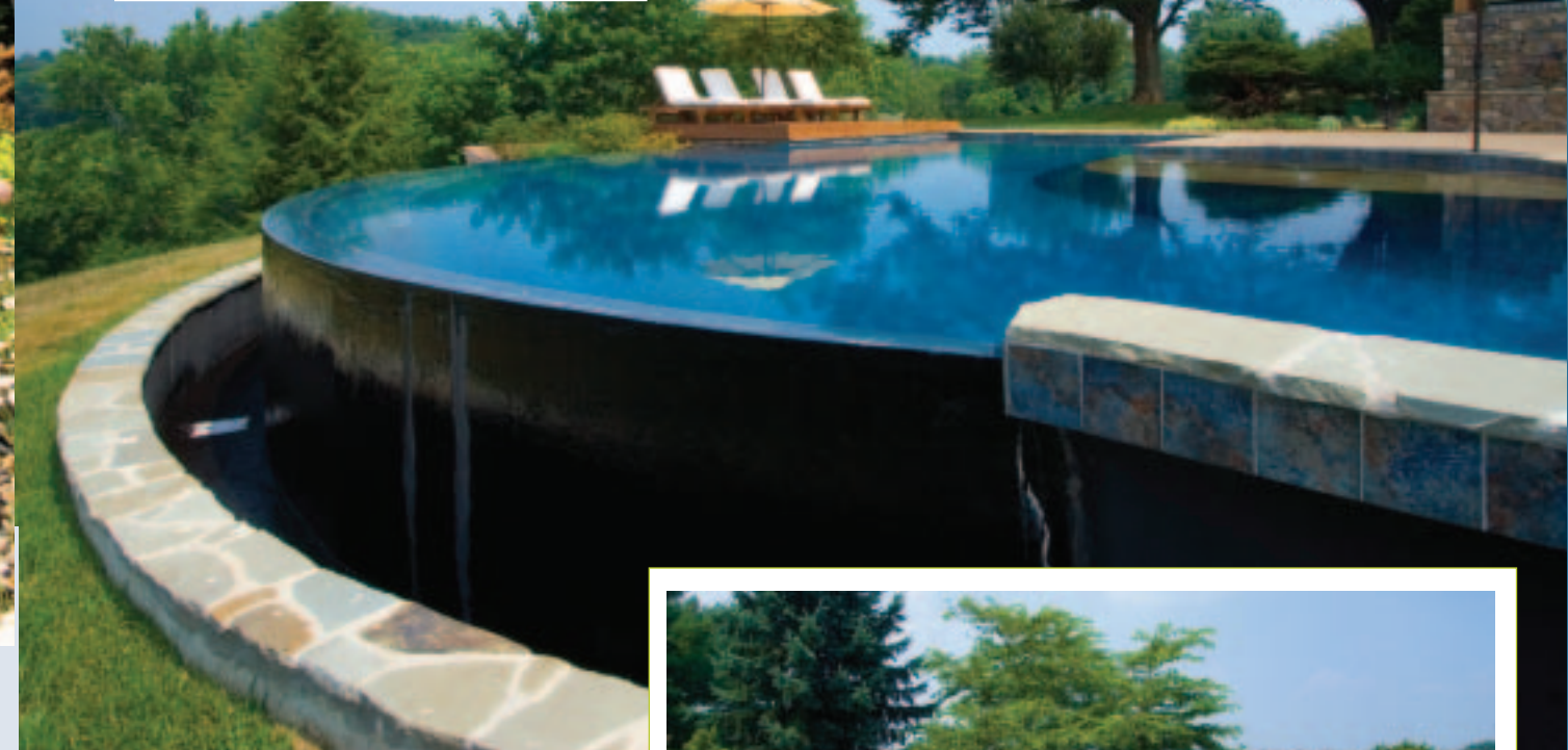
To create the pool's negative-edge effect, water flows over the circular rim and into a catch pool below. (top) A soothing waterfall flows from a stone wall into a raised spa situated to one side of the pool. (cover photo) An Ipe wood deck to the right of the pool's entry offers the perfect spot to enjoy the sun and breathtaking hilltop view.
